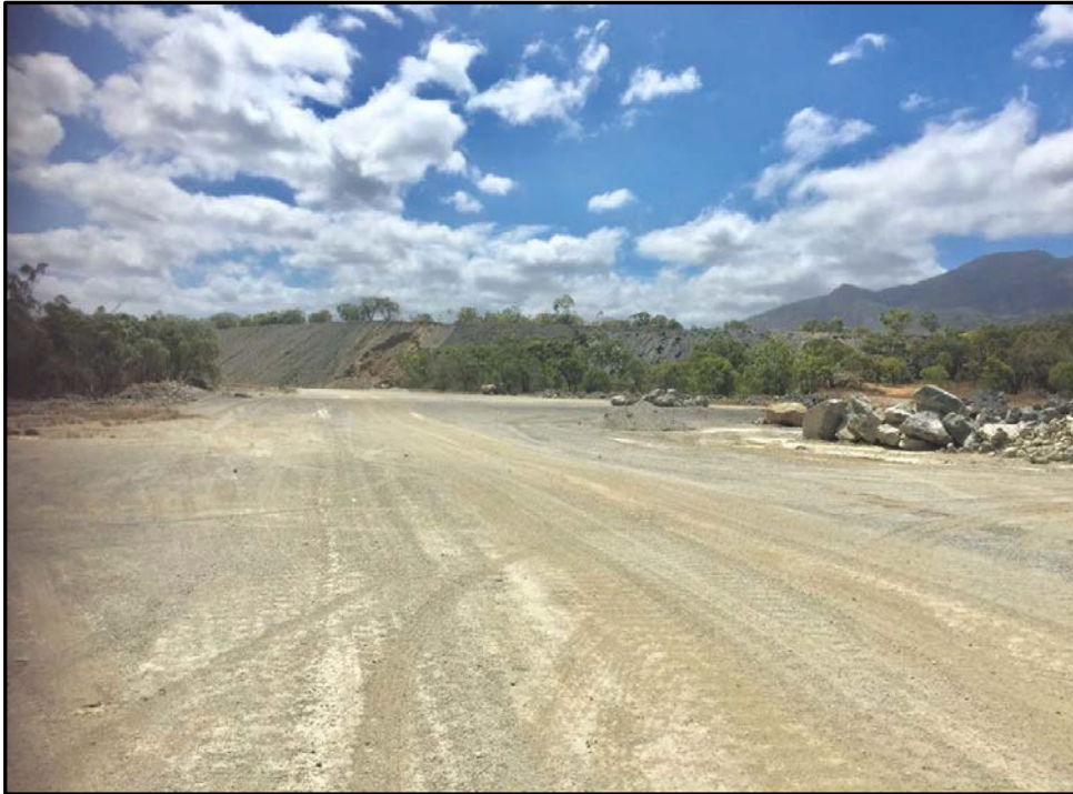
Figure 1-4: Mt Carbine Site Haul Road
