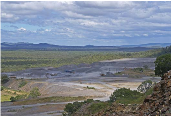
View from the top of the pit to the stockpiles.
