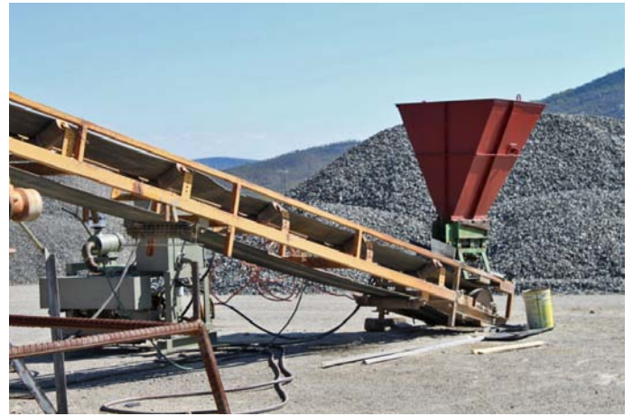
The feed hopper and conveyor to the X-ray ore sorter.
