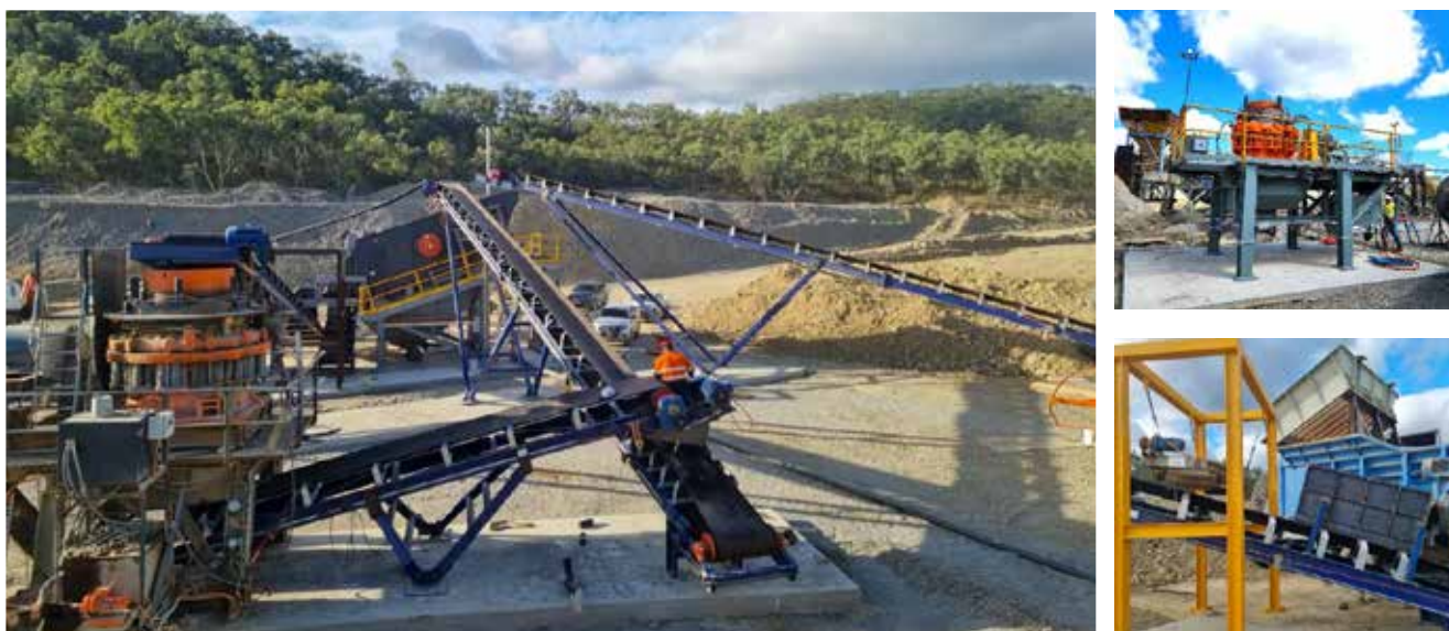
Newly installed screening and crushing plant.
