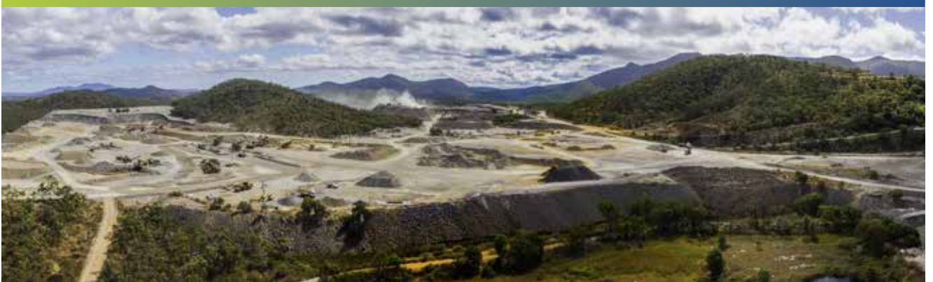
Mt Carbine Low Grade Stockpile and Quarry Operations
