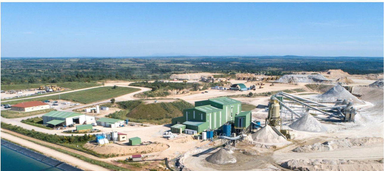
Saloro's Barruecopardo mine in Spain, with the processing plant on the left and crushing and screening circuit on the right.
