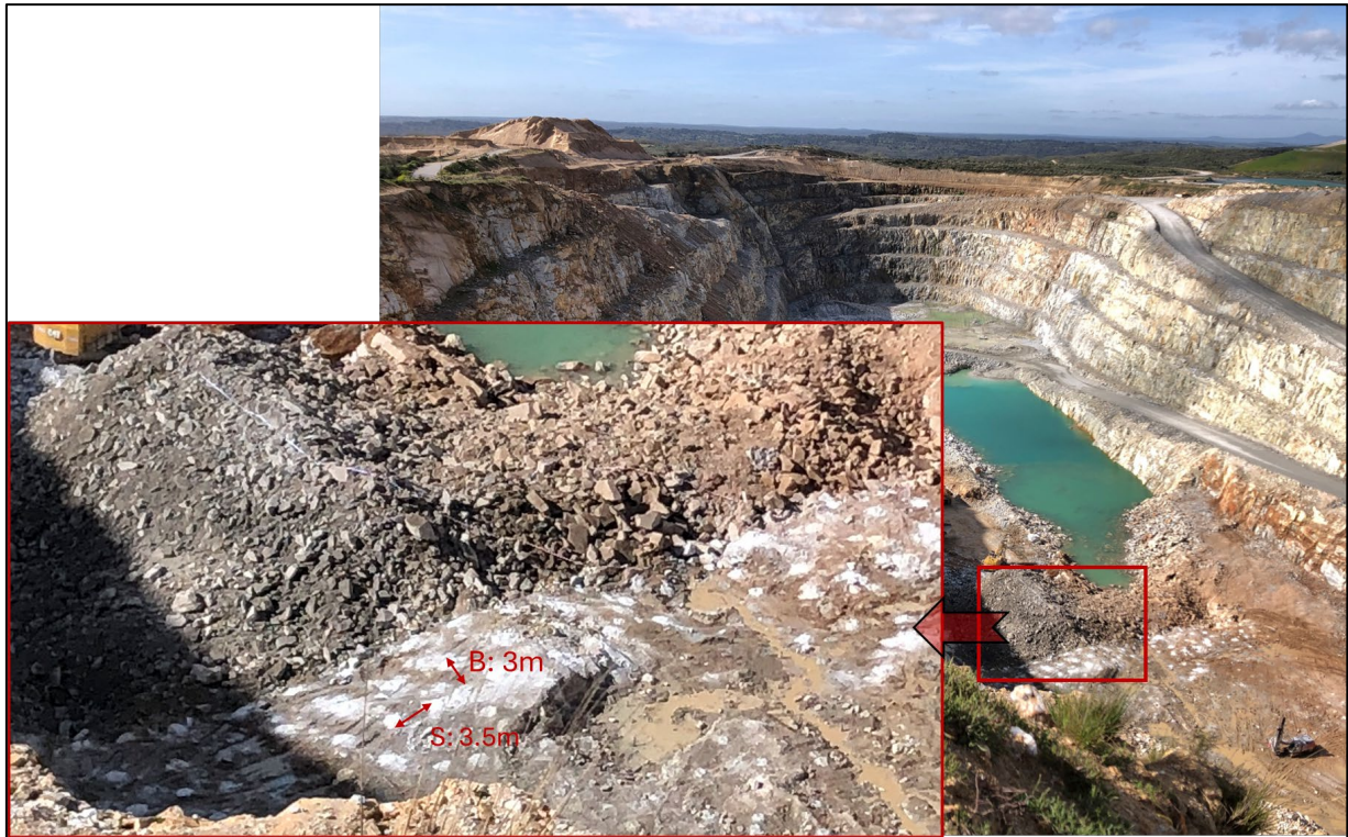
Figure 7-4 Blasting area in the bench 590. April 2024
