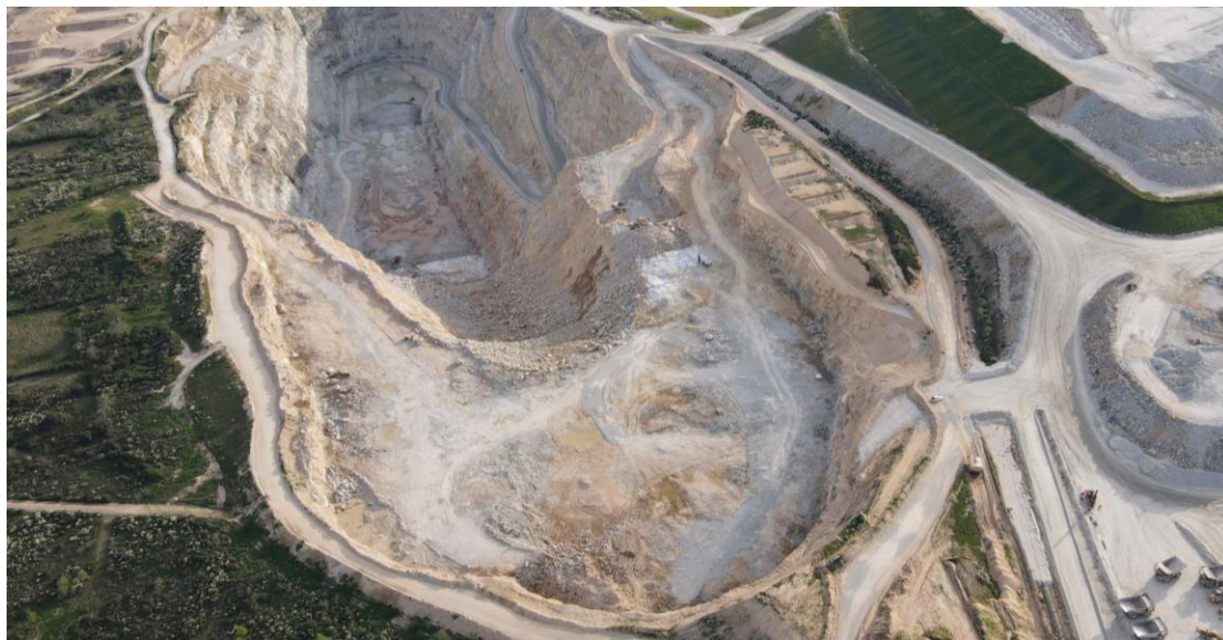
Picture above: Northern area of Phase 6 Pit at level 700 RL looking South, including the access ramp and bench at level 690 RL, with ore stockpile on the front left and waste dump at the back as of the end of March 2025.
