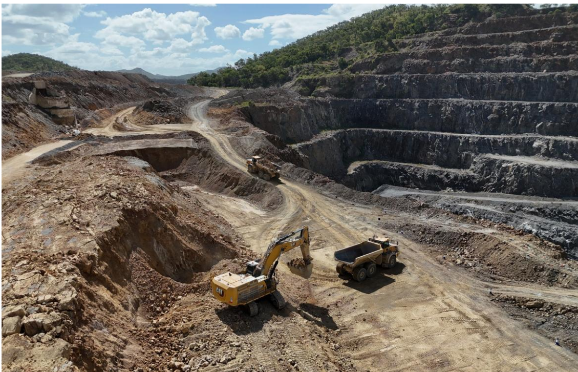
Picture above: CAT 320 Excavator and Volvo 60 tonnes Articulated Dump trucks in the South Area at level 375-365 RL
