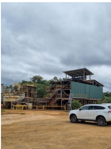
Figure 3: Gravity plant at Wolfram Camp.
