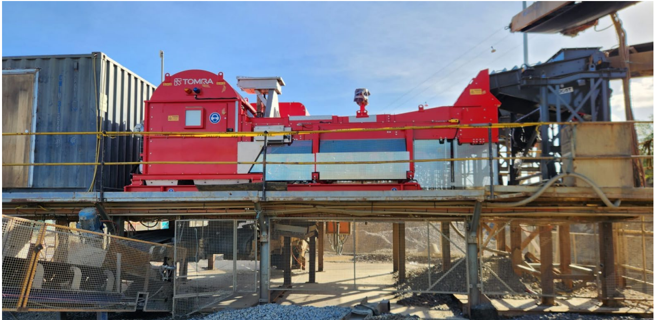
Figure 9: The New TOMRA 3 XRT Sorter is installed and being commissioned.
