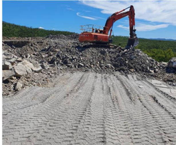
Figure 1 - Stockpile truck loading ramp
