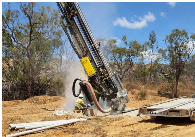
Drill rig operating in the eastern extension.
