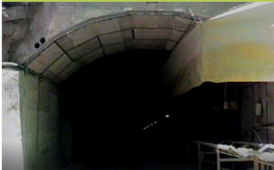
Mt Carbine Existing Decline - Historical Pictures 1986
