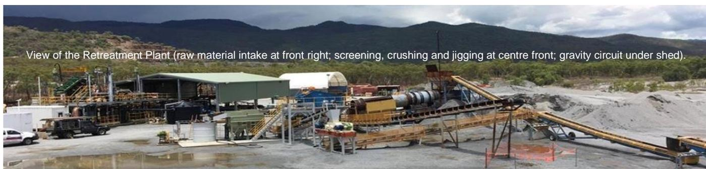
View of the Retreatment Plant (raw material intake at front right; screening, crushing and jiggling at centre front; gravity circuit under shed).
