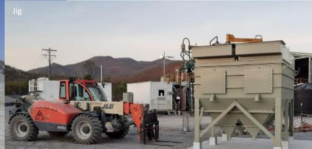
Steel support structures & equipment positioned in preparation for electrical installation and commissioning.
