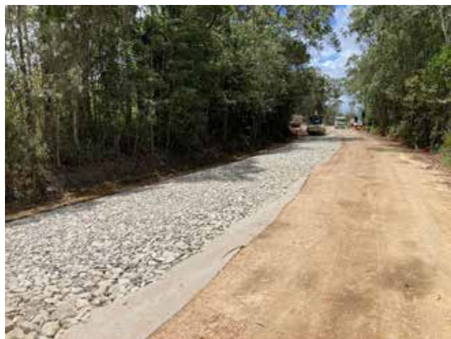
Euluma Creek Roadworks.
