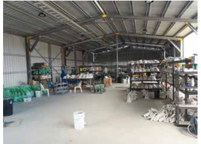
Newly constructed laboratory and core shed.
