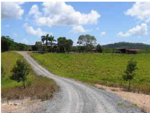
Julatten Road Rebuild.
