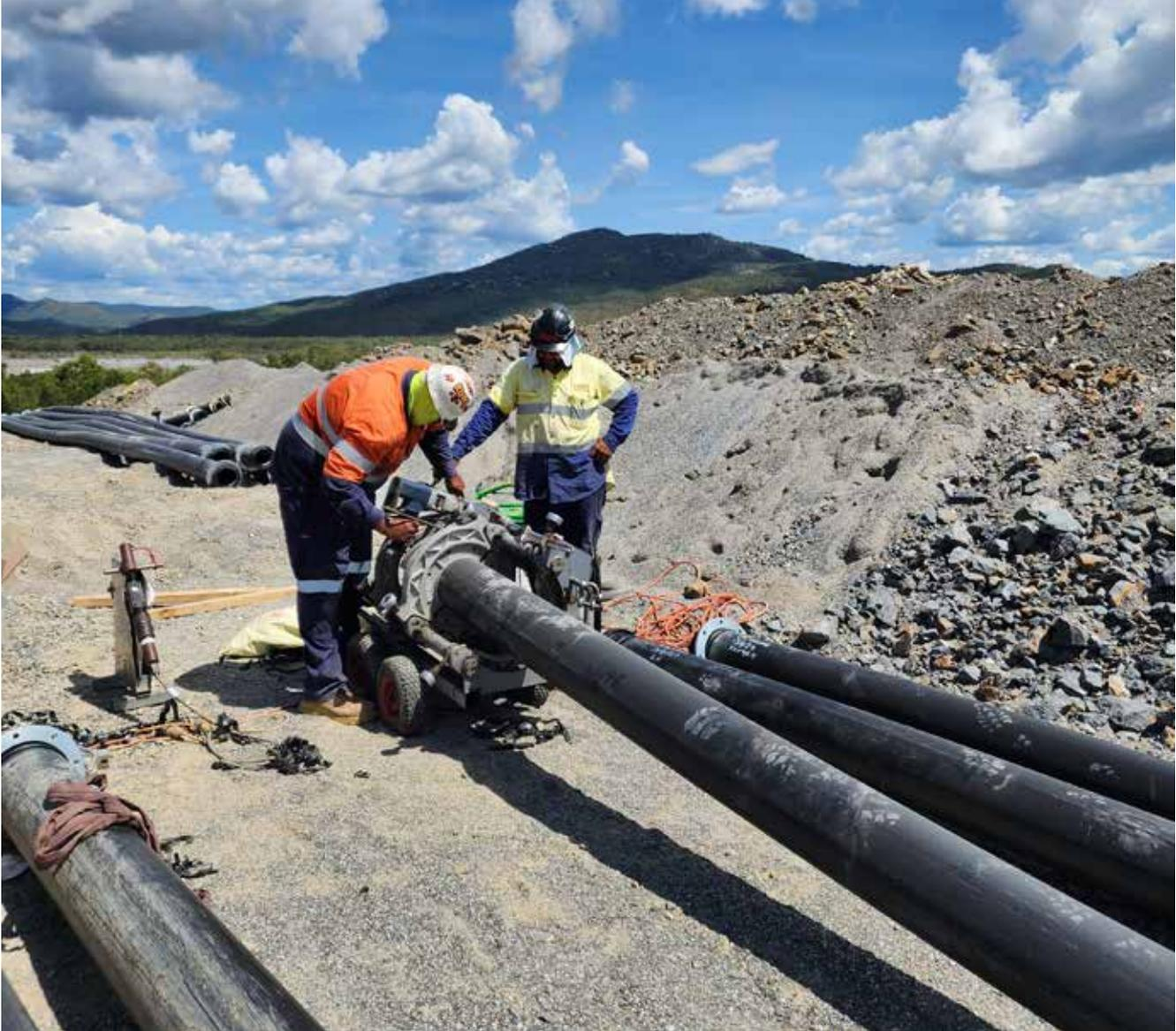
Efficient transportation of fines from the crushing Plant to the Gravity Plant has been achieved through the successful implementation of slurry lines.
