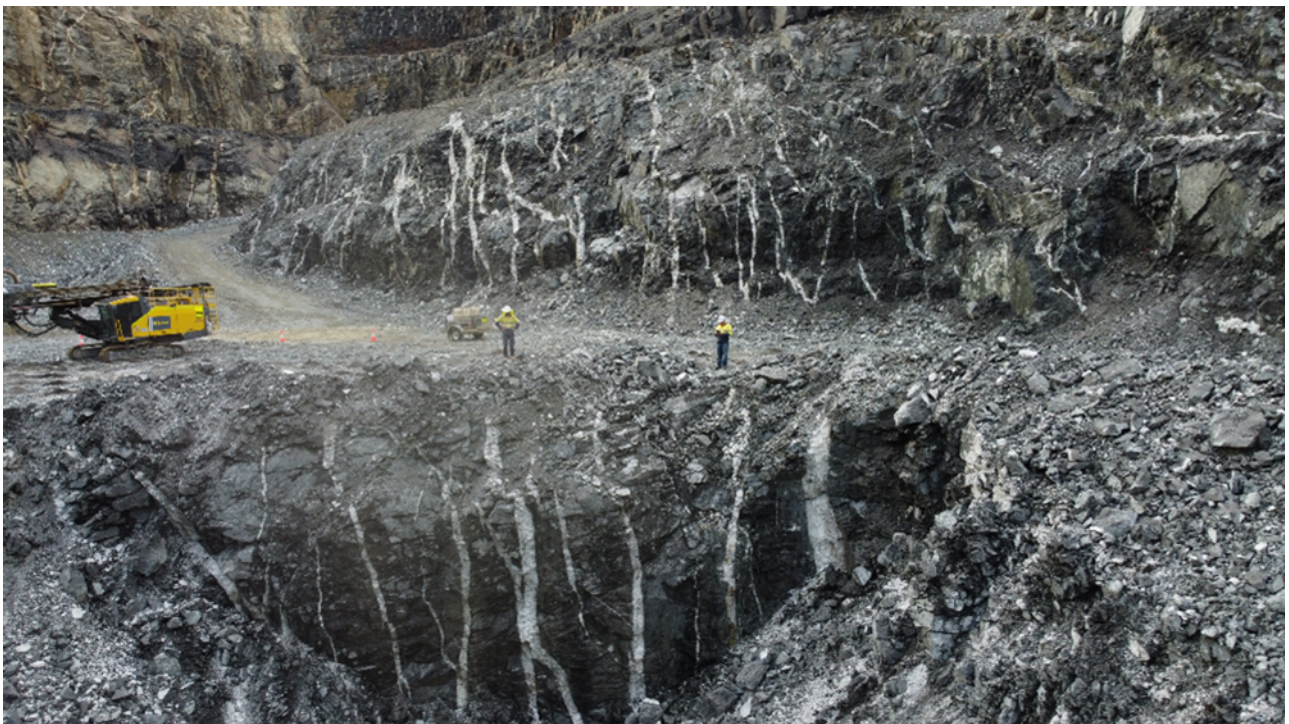
Fig. 4 - Picture showing the continuity of the veining in open pit, tests are planned to follow some of these veins underground
