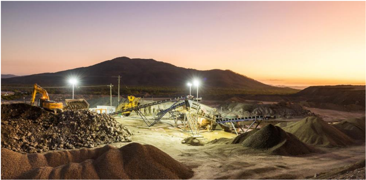
Figure 2: Upgraded Crushing and Screening Area – Completed in Phase 1
