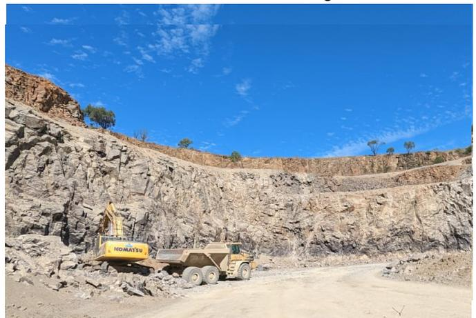
Fig. 1 - Earth works and preparation of pit ramp
