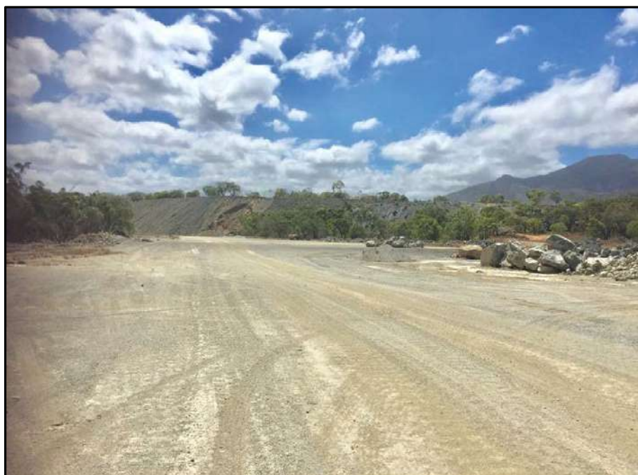
Figure 1-4: Mt Carbine Site Haul Road
