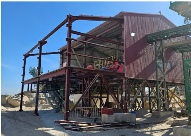
Picture left: the Ore Sorter Plant shed being extended to make room for the third Ore Sorter. Picture right: the Wet scalping screen being installed in front of the Ore Sorters
