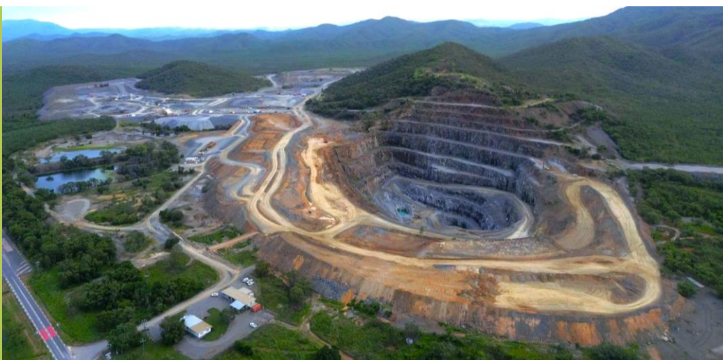
Mt Carbine Open Pit & Processing Plants
