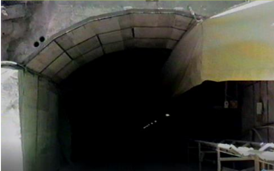
Mt Carbine Existing Decline - Historical Pictures 1986
