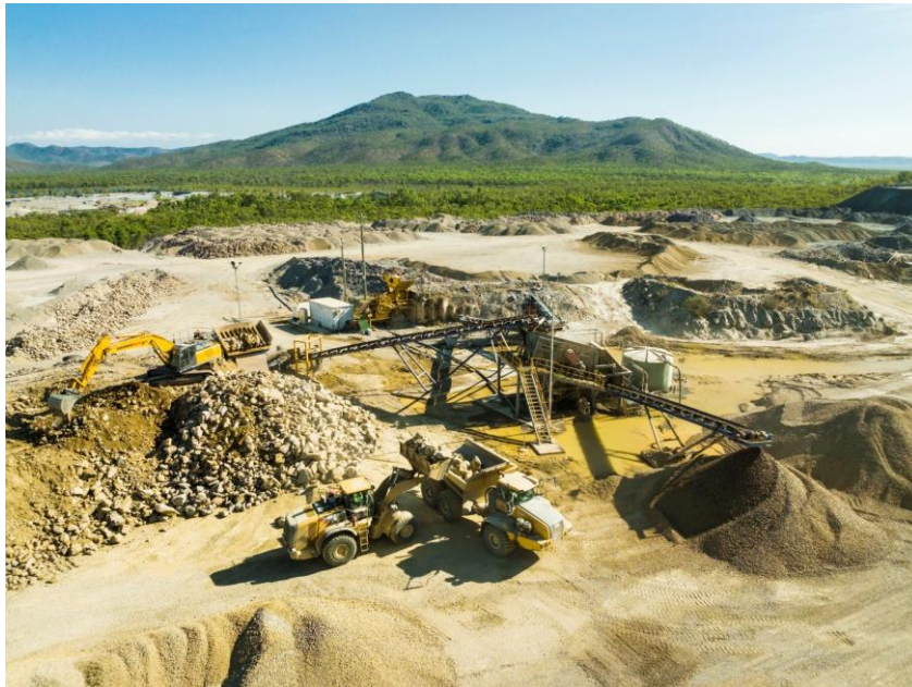
Figure 1 - Crushing plant achieving throughput targets.
