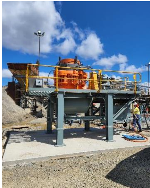
Figure 2 - Tertiary Cone Crusher for XRT Sorter Concentrate
