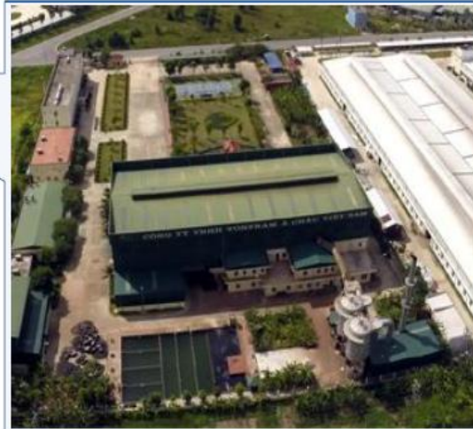
TMG Ferrotungsten Plant
