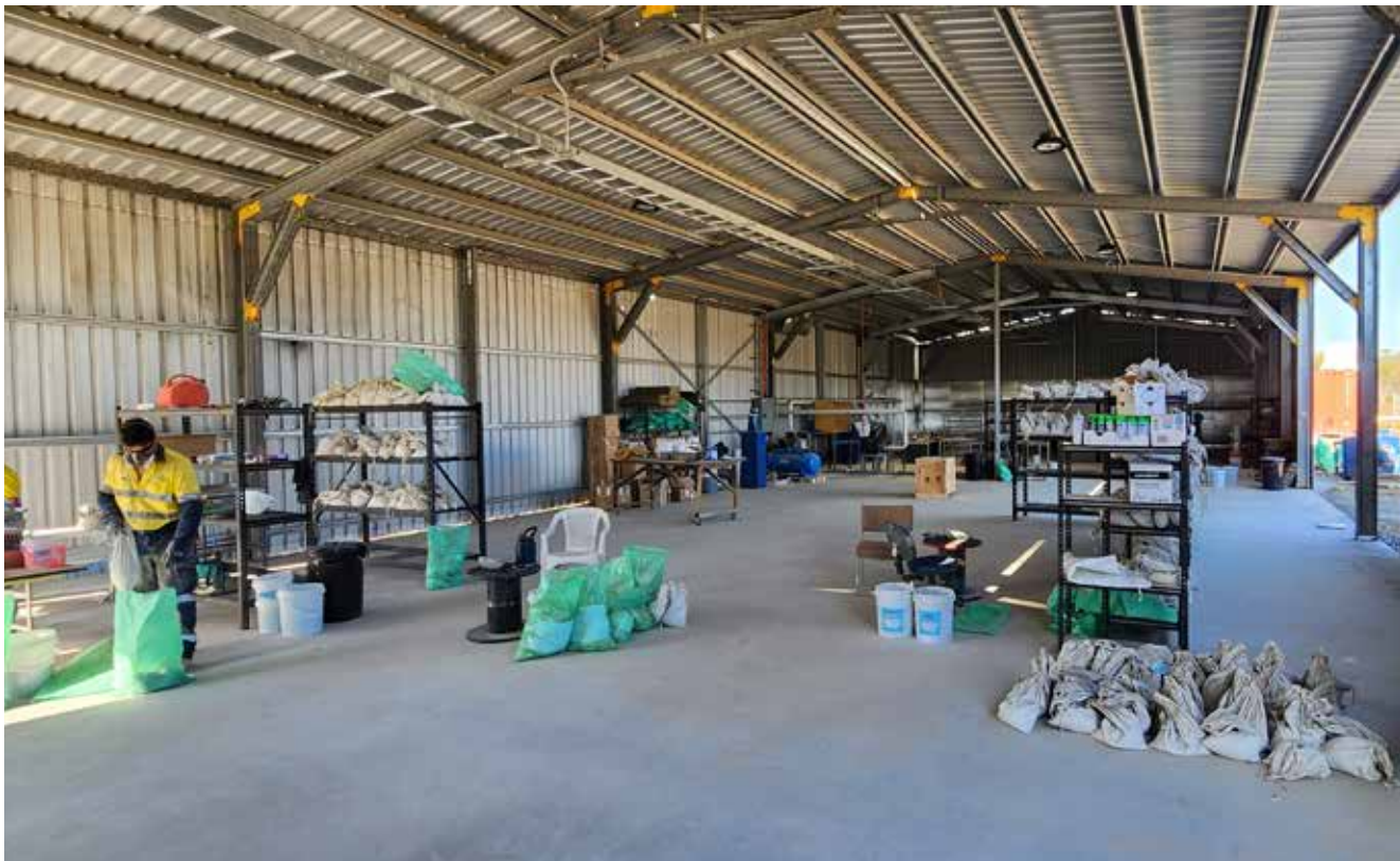
The newly established laboratory shed before all equipment and shelving was put into place.
