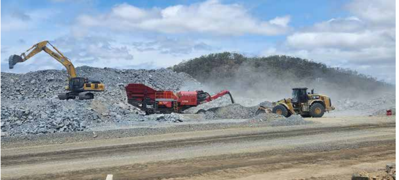
Kobelco 50 tonne excavator feeds the newly commissioned Terex Finlay Jaw Crusher J-1175 before the CAT 980M Front End Loader transports the feed to ROM1 Stockpile for the Crushing Plant.
