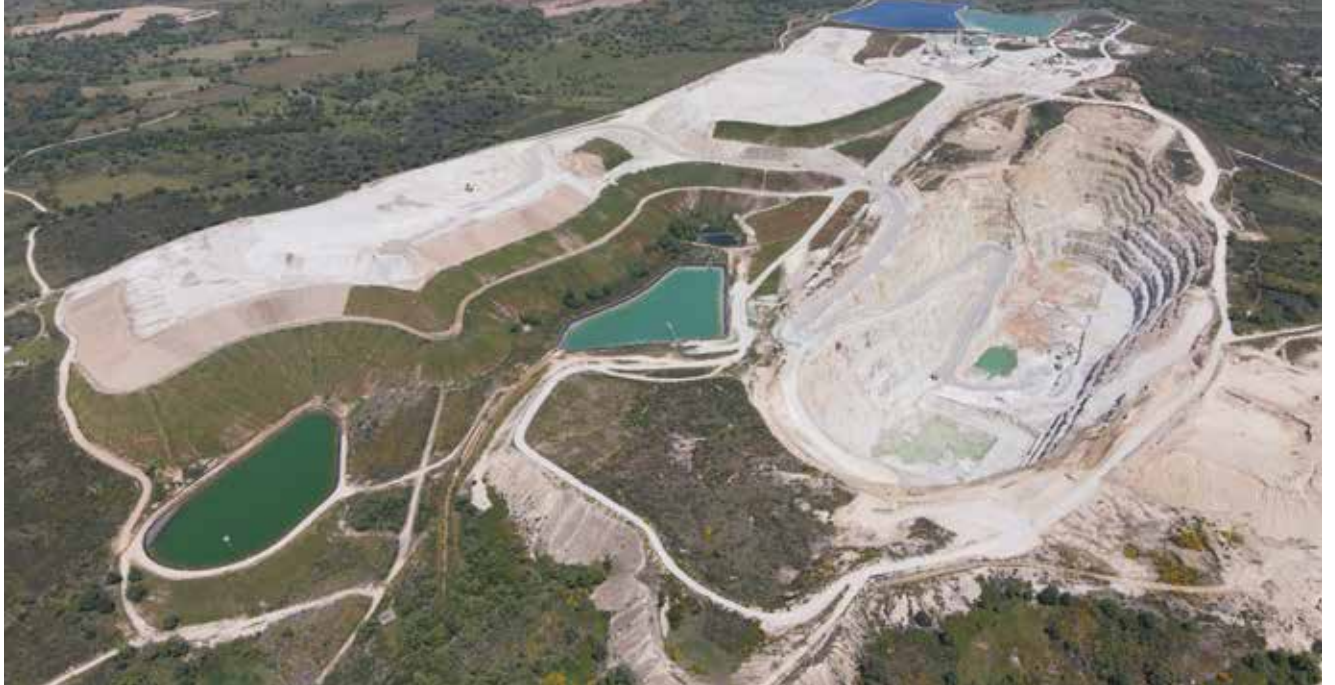
Barruecopardo Open Pit as of end of June 2024.
