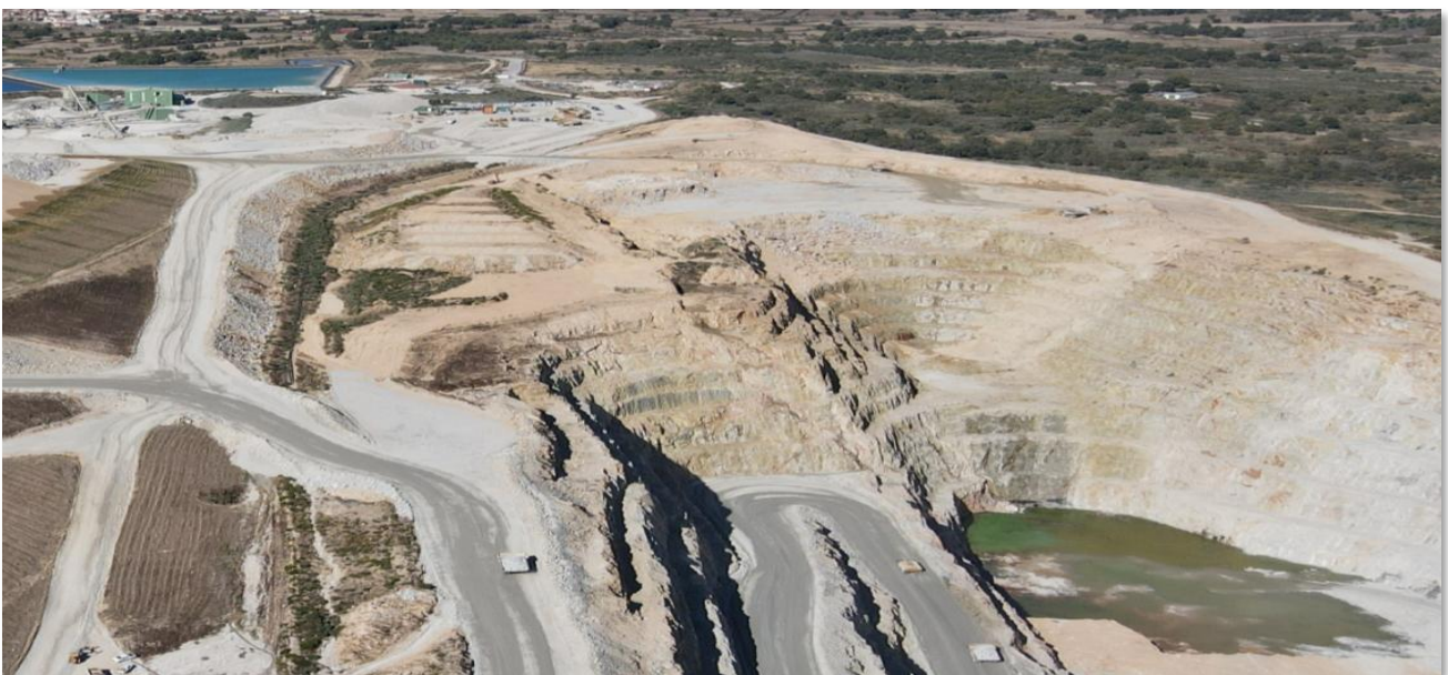
Pictured: The Northern Area will be the target of Phase 6, next phase of the Open Pit.
