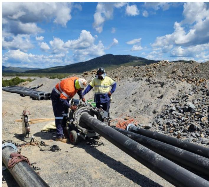
Figure 4 – Upgrading of slurry pipeline.
