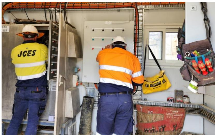
Figure 3 – Electricians installing PRC wiring for automation control on the crushing circuit.
