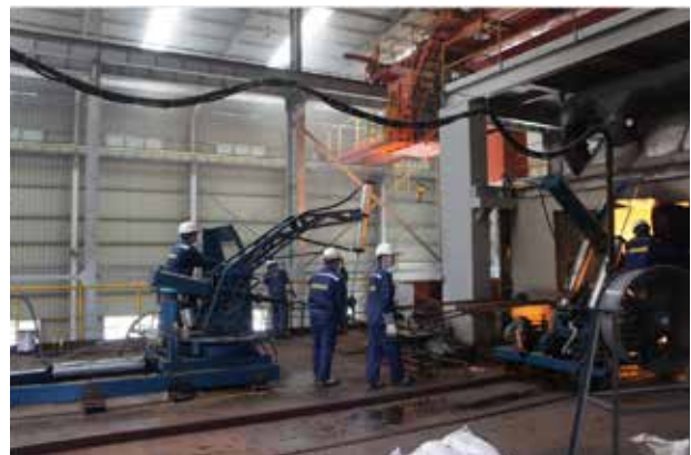
Pictured: the TMG ferrotungsten plant located in Vietnam. Source: ( www.tungstenmetalsgroup.com )
