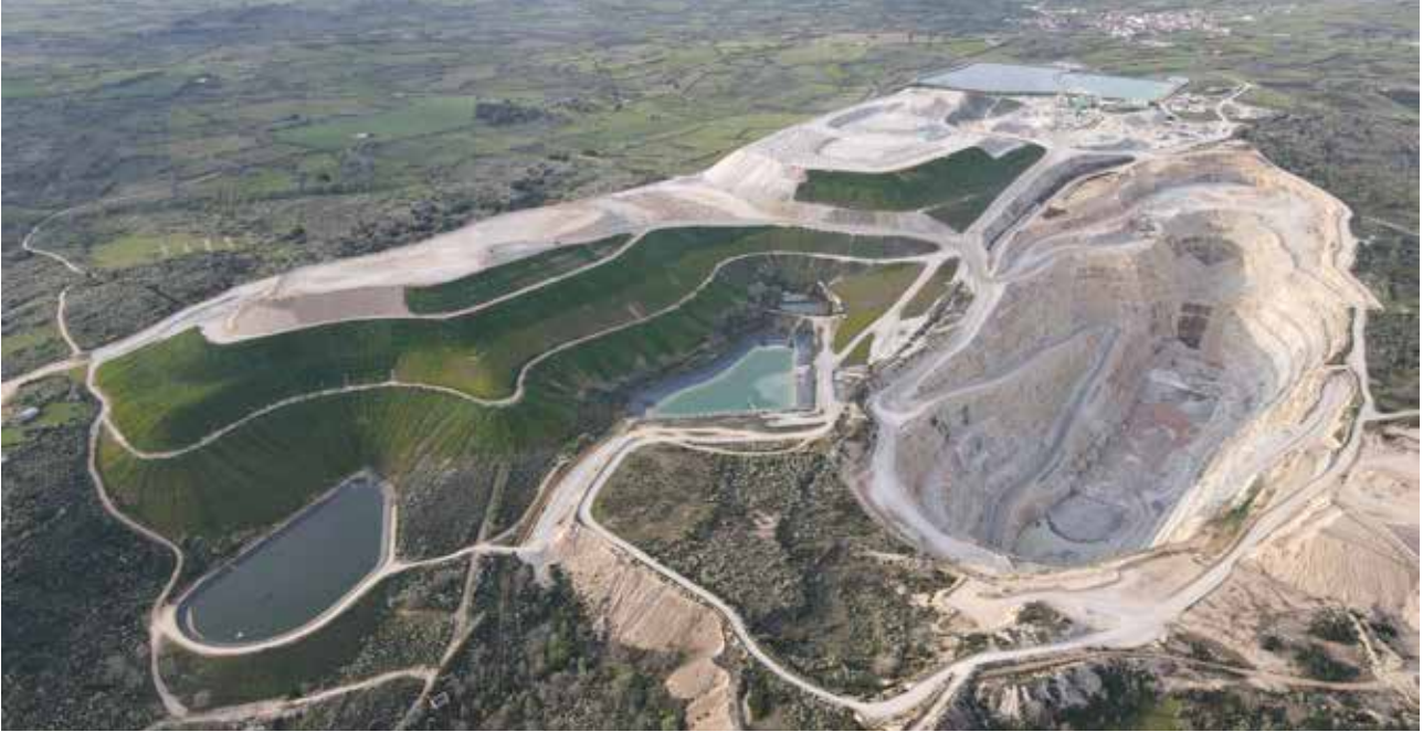
Picture above: The Barruecopardo Mine Open Pit as at March 2025 looking north, with ongoing progressive rehabilitation of the waste dumps near the water dams on the front left.
