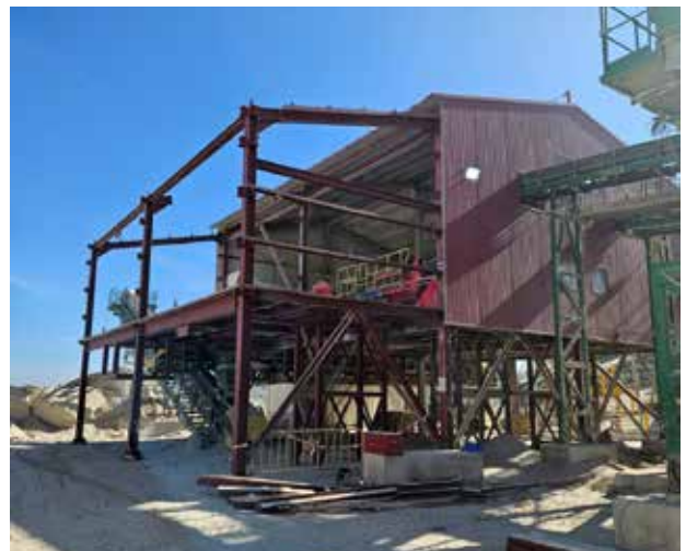
Pictured above left: the Ore Sorter distribution hopper installation progressing. Picture above right: the existing building containing the two ore sorters being extended to make room for the third ore sorter.
