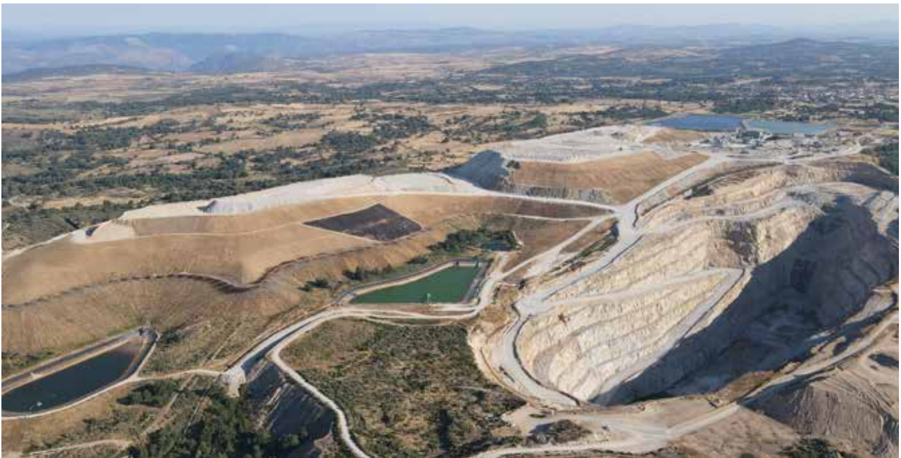
Picture above: The Barruecopardo Mine Open Pit (Spain) at the end of June 2025.
