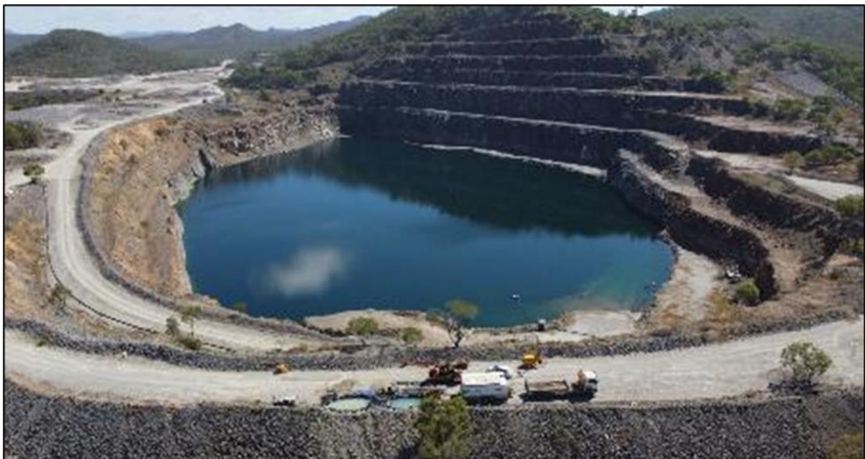
Figure 3-1: Current Pit Showing Historical 20m Benches
